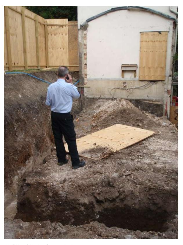
Plate 5. Foundation trenches completed
