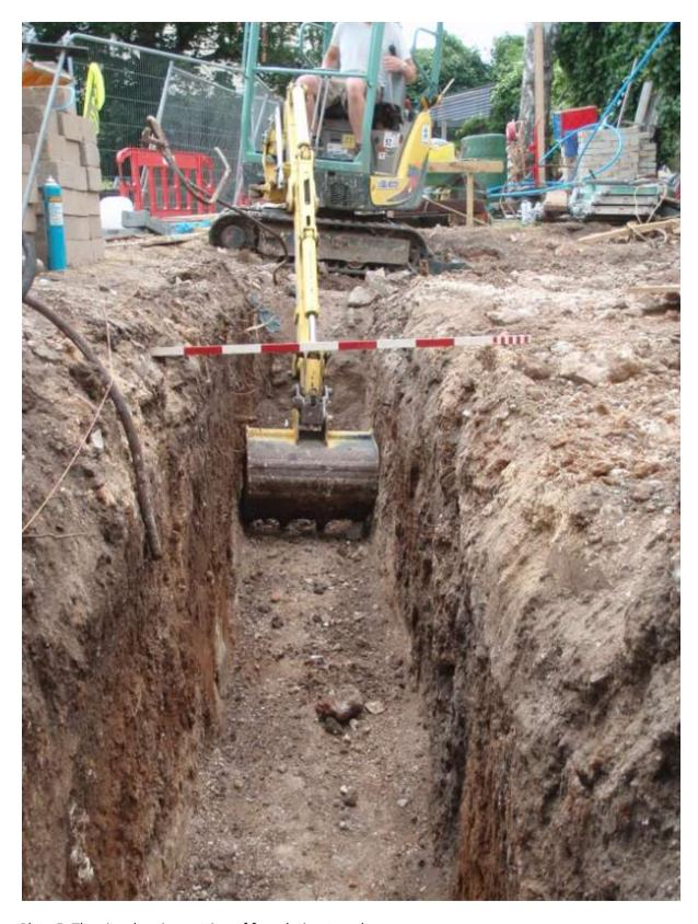
Plate 5. The site showing cutting of foundation trenches
